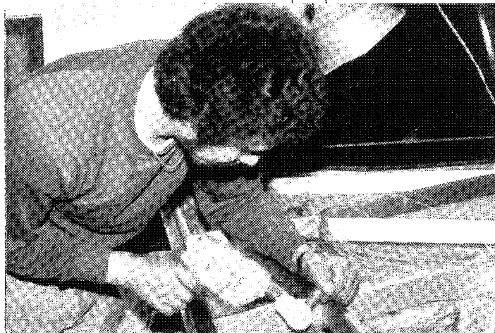
A series of holes must be drilled to fill the crack with threaded studs.
